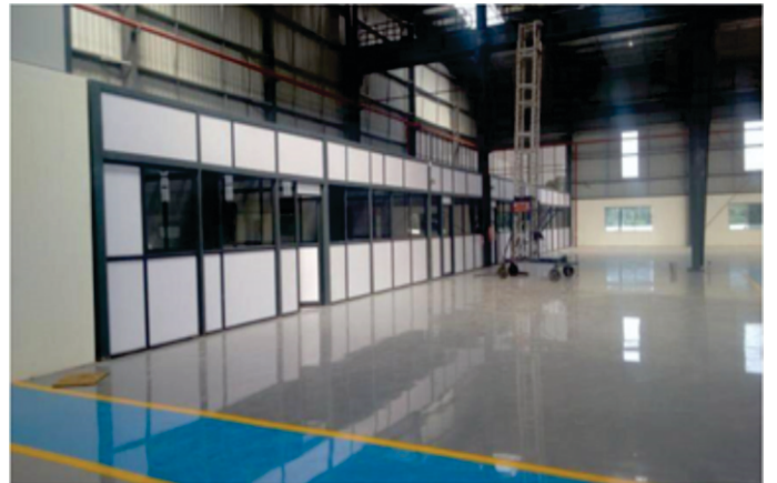
M/S Shree Motherplast Pvt Ltd (Vallam-Chennai) Office Area Partion Work
