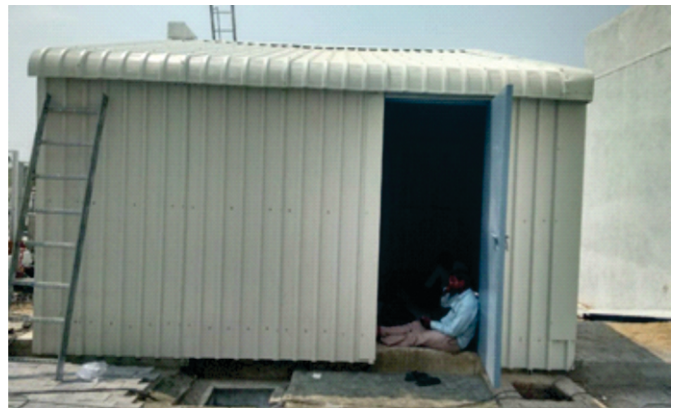
M/S RUHRPUMPEN India Private Limited (Vallam-Chennai) Electrical Panel Room Shed Work
