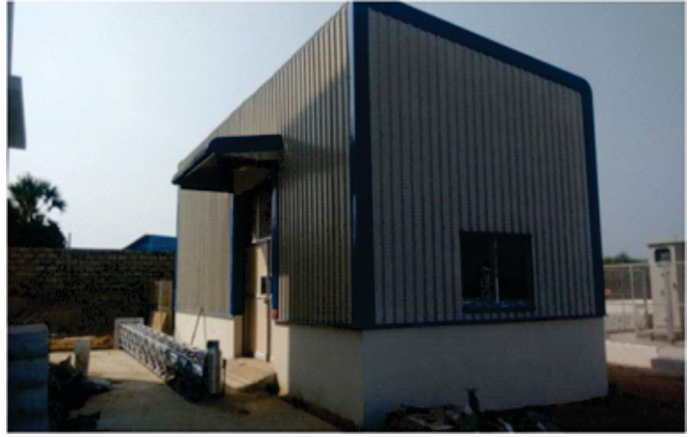
M/S Shree Motherplast Pvt Ltd (Vallam-Chennai) Electrical Panel Room
