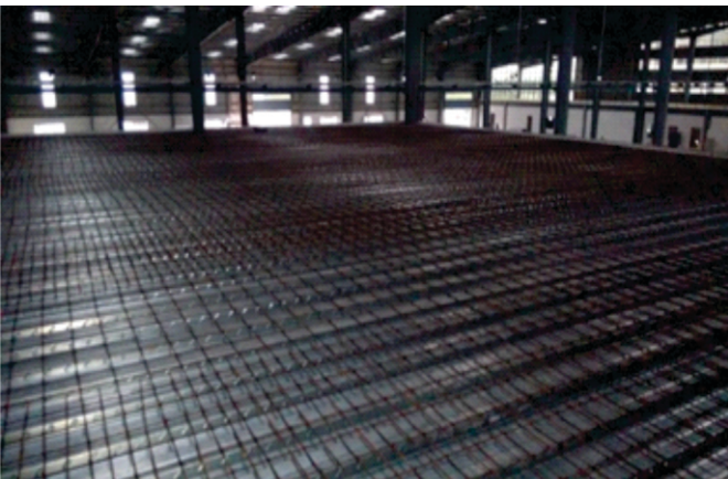
M/S Asian Sealing Products Pvt Ltd (Pillaiakkam-Chennai) Deck Slab Work
