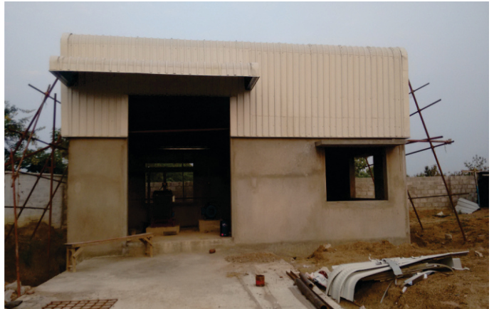
M/S Asian Sealing Products Pvt Ltd (Pillaiakkam-Chennai) UG Sump & Pump Room
