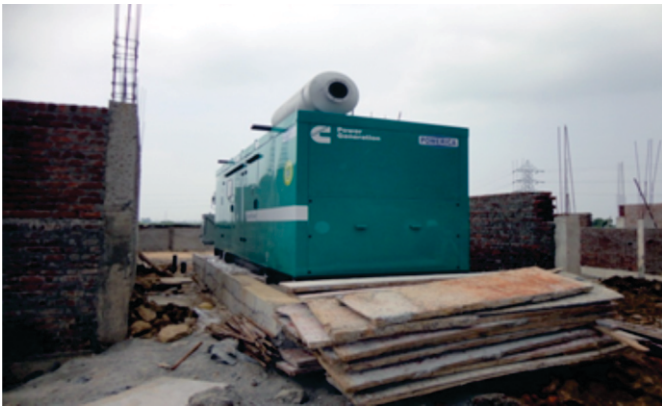
M/S Varroc Polymers Pvt Ltd (Oragadam-Chennai) DG Bed Foundation Work
